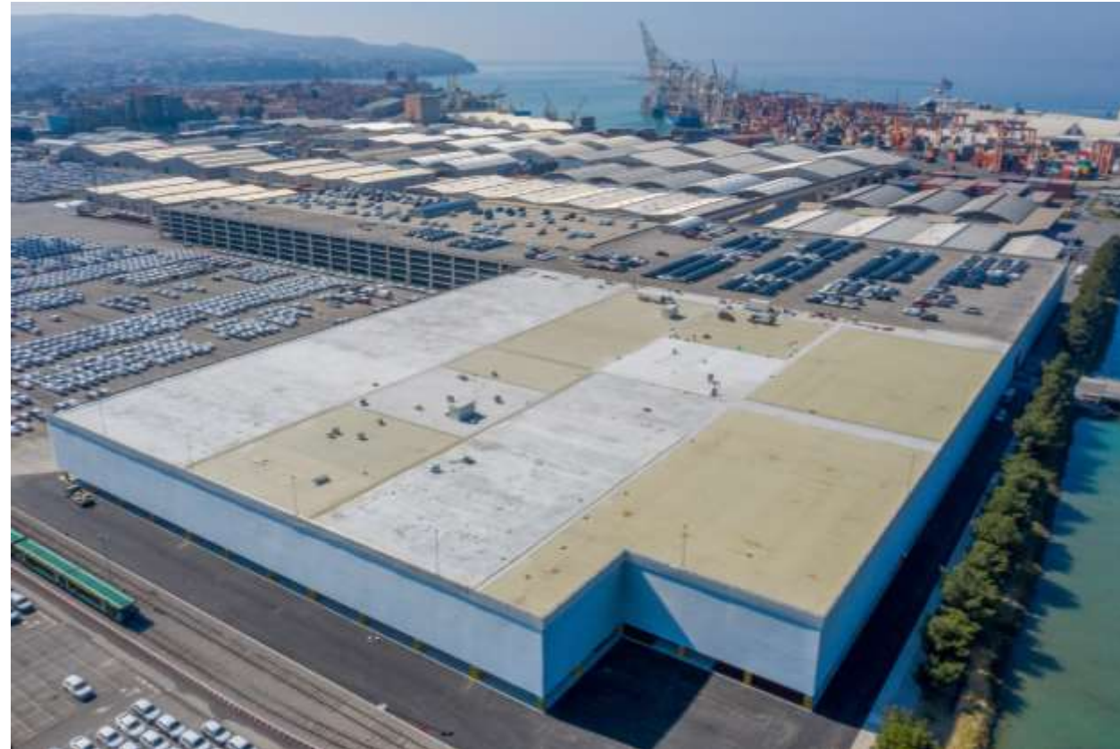
New garage building with 6.000 parking lots
