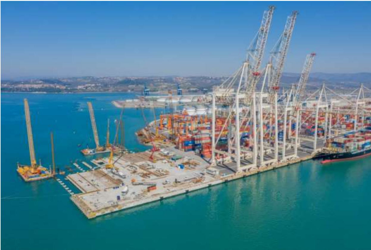
Extension of container quay
